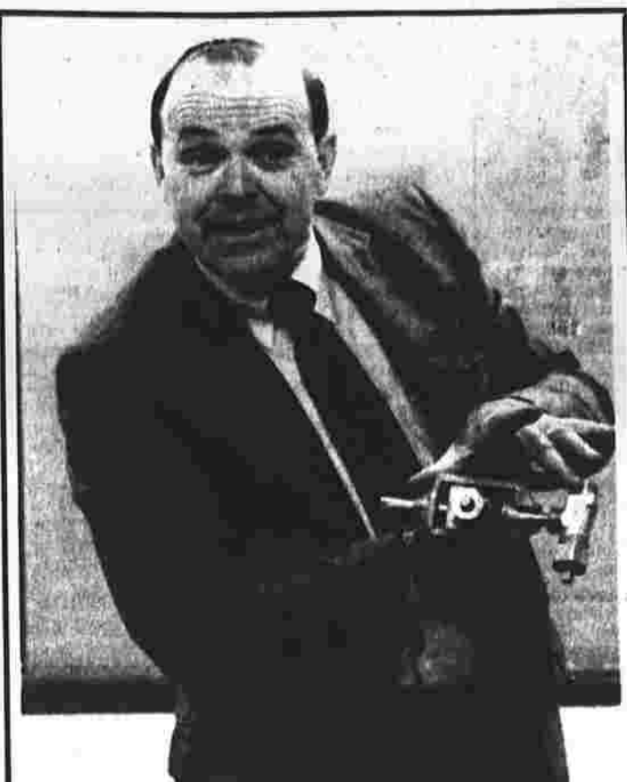
John Day Jr. of the Hubbard-Hall Chemical Co. shows workers how to plug a leak at the Globe Hollow water treatment plant on Spring Street.
